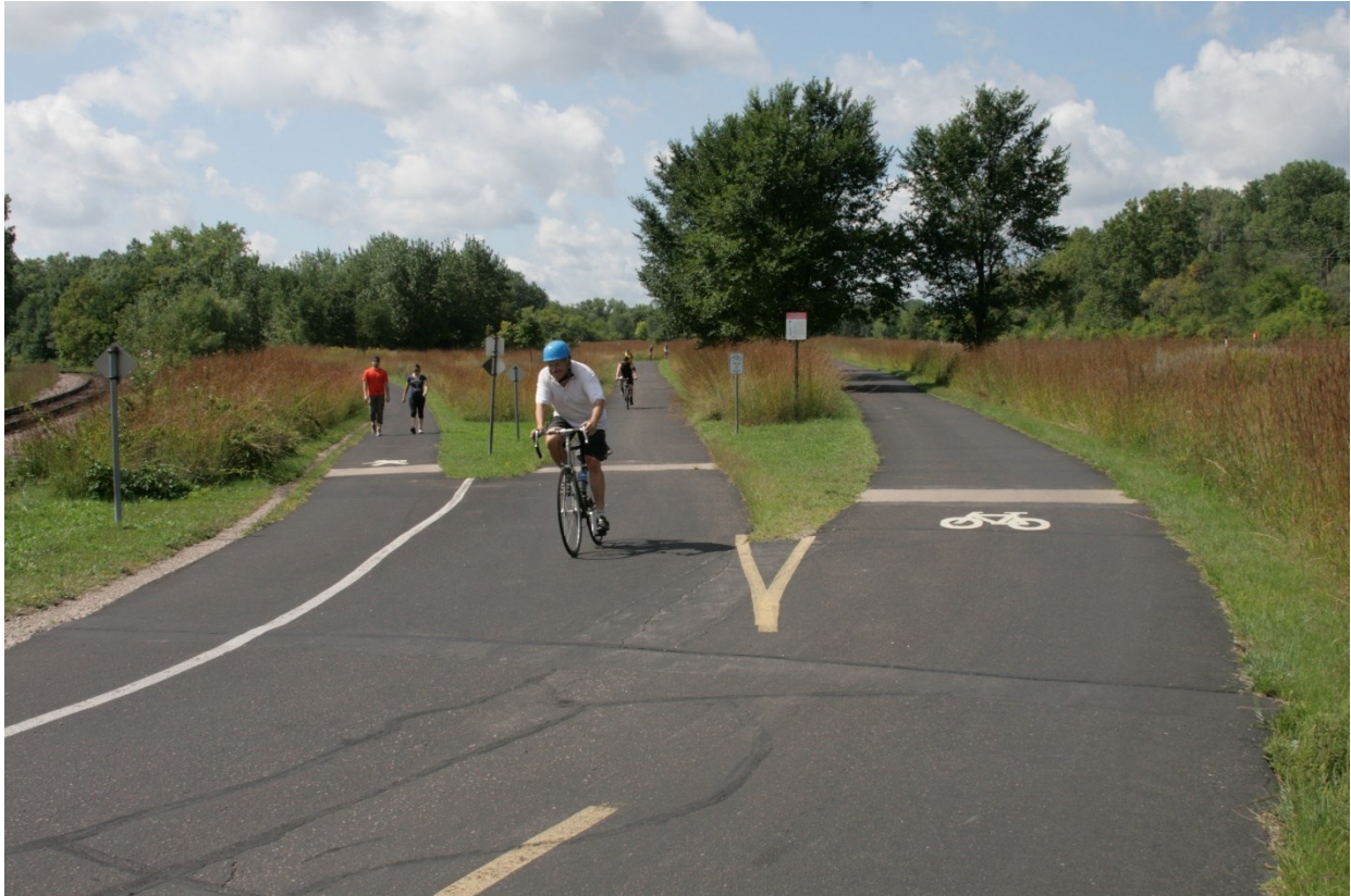
Figure 12: Shared-Use Path in Minneapolis, MN Source: Toole Design Group
