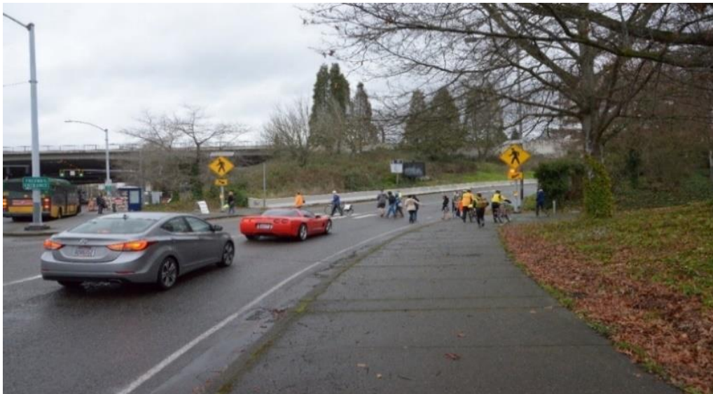
Figure 12. The conditions at this I-90 on-ramp from Rainier Avenue South illustrate what pedestrians have been facing in the area around the future light rail station and in other locations across the state. With designs like this, people have to cross at a point where drivers tend to accelerate to highway speeds.
