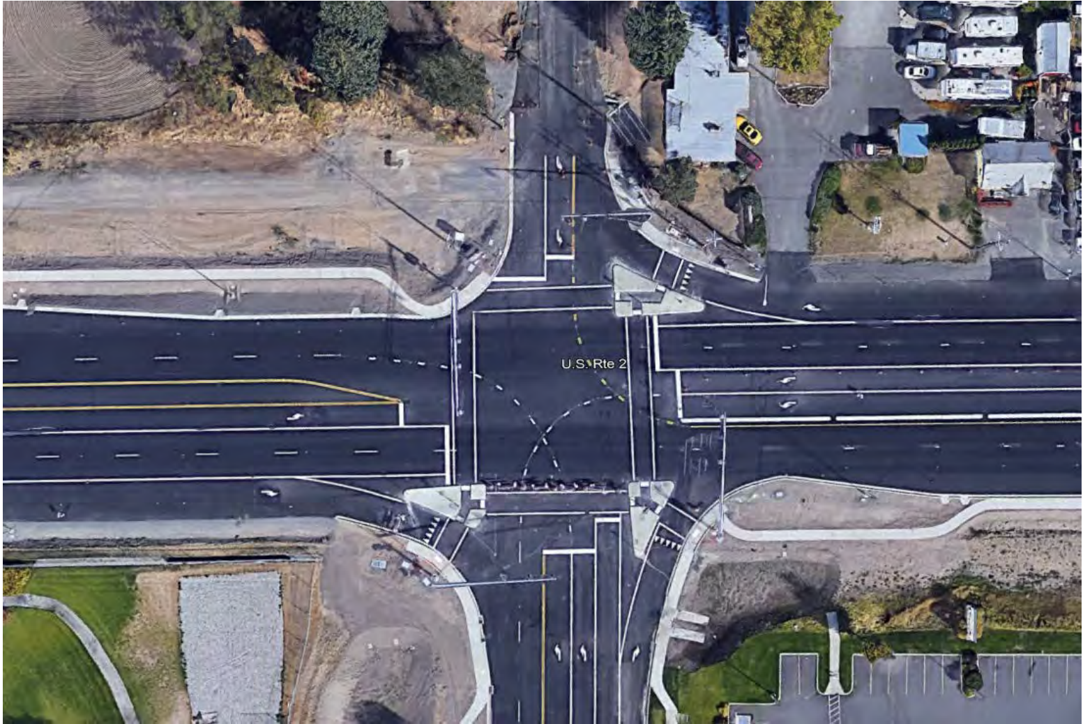
Signal Installed Sept of 2014
